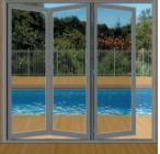
Left: Although this 145Kg home spa pool door is operated successfully with a SelfLatch/SelfClose system, doors heavier than this can present challenges. Similarly, self-closers are impractical for bifold doors, especially if the passage door is hinged on a folding section. DoorMinder alarm systems offer effective home-pool safety solutions for both, with innovative componentry concealed within the door-frame.
