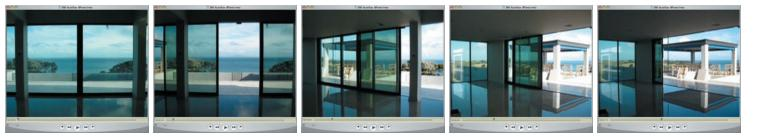
**One side of the story:** The motion of four of the eight panels in this 16-metre bi-parting door-set are tracked in a vid-cam sequence during initial trials. This AutoStac R500 installation is regarded as the largest of its type in Australasia and a first for a residential site.
