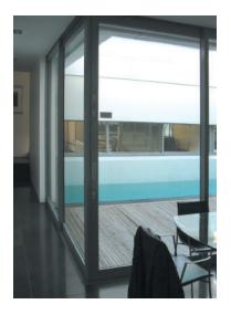
This angled sliding door configuration makes the most of linking pool zone and interior. The Swish SelfLatch/ SelfClose system is concealed in the right slider panel. In the closed position. the left slider is immovable, and remains so even when the right panel is opened to access the pool zone.
