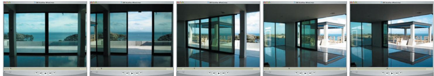
*One side of the story: The motion of four of the eight panels in this 16-metre bi-parting door-set are tracked in a vid-cam sequence during initial trials. This AutoStac R500 installation is regarded as the largest of its type in Australasia and a first for a residential site.*
