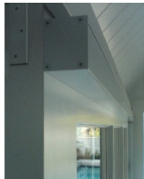
*Left: Tidy solution for a challenging timber sliding door arrangement: End view of the surface-mounted duct concealing a SelfClose™ system.*
