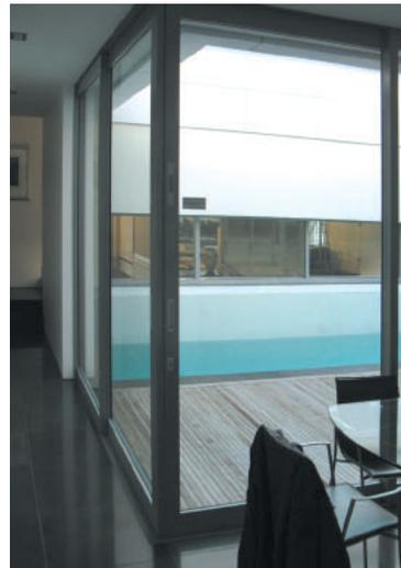
*This angled sliding door configuration makes the most of linking pool zone and interior. The Swish SelfLatch/ SelfClose system is concealed in the right slider panel. In the closed position, the left slider is immovable, and remains so even when the right panel is opened to access the pool zone.*
